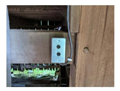
To turn the power off, press and hold the bottom button for at least 10 seconds. You should hear the inverter whine and the pitch drop. DO NOT RELEASE THE OFF BUTTON UNTIL THE WHINE STOPS!!!! Even though the lights should turn off immediately, the inverter can turn itself back on until the output charge dissipates.
