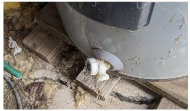
• Access/Relief valves in water heater shed. Turn these off by turning the handles in the clockwise direction.
